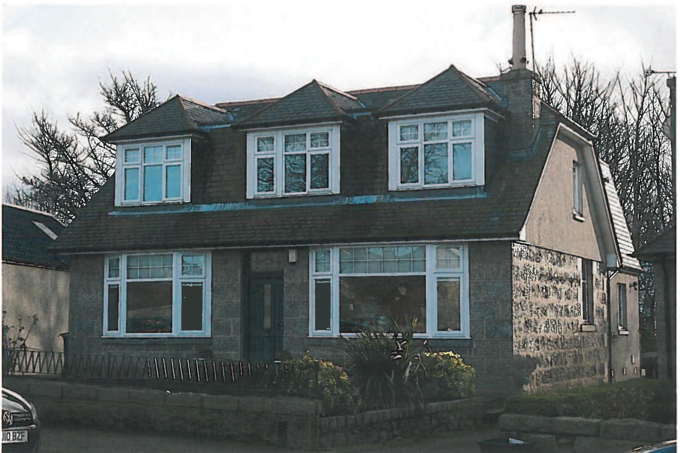
8. DETACHED DWELLING - GABLED - KING'S CROSS ROAD
