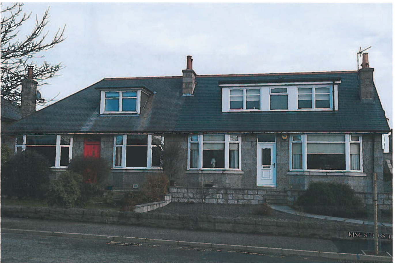
6. GABCE CONVERSION 2 - FRONT
